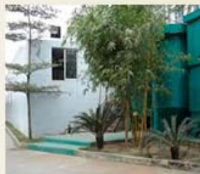
Water Treatment System
